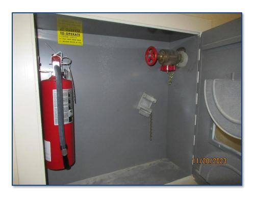
Photograph No. 34: Fire extinguisher and fire hose valve.
