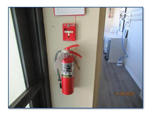
Photograph No. 33: Fire extinguisher and fire alarm pull station.
