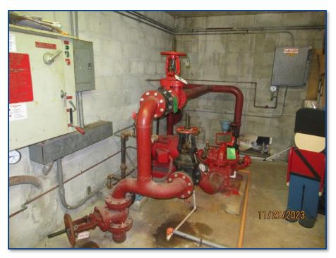
Photograph No. 35: Fire pump motor and valves.
