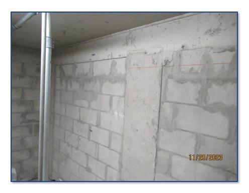
Photograph No. 29: View of the concrete masonry unit walls, concrete column, and concrete beam.
